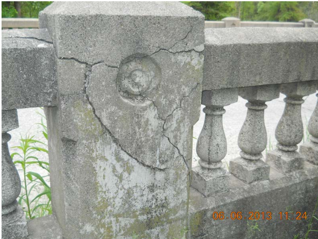
Delaminations, wide cracks on barrier post.
