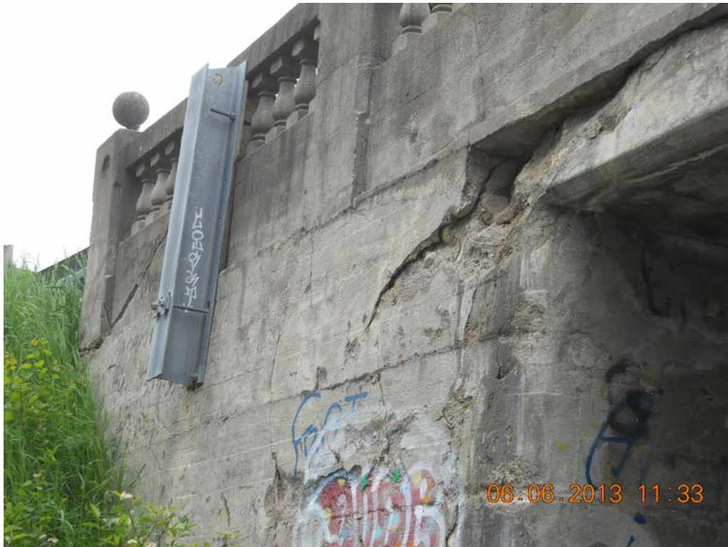
Spalls, delamination on wingwall and fascia.
