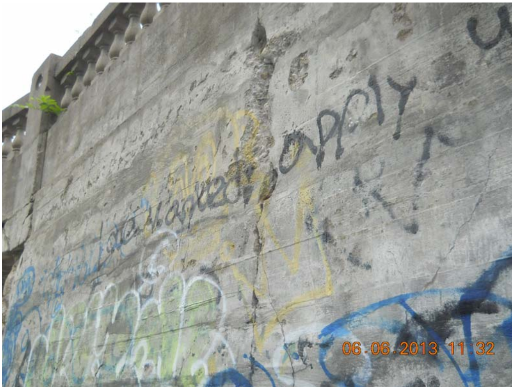
Spalls, wide crack on wingwall.
