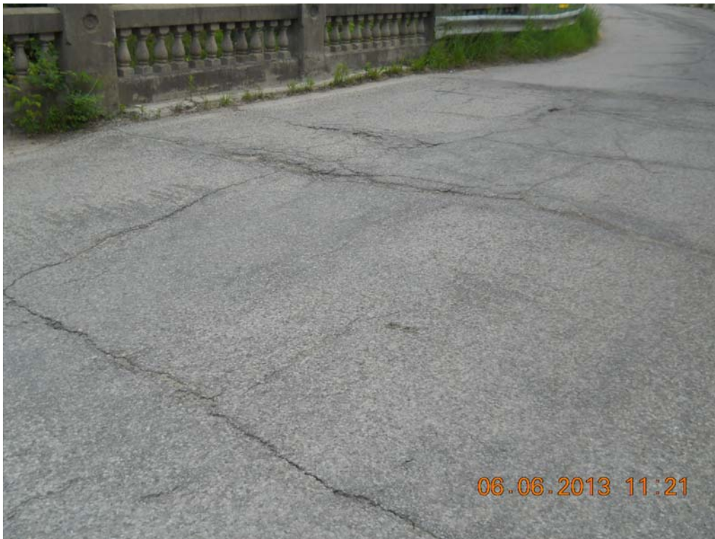
Narrow to wide cracks on wearing surface.
