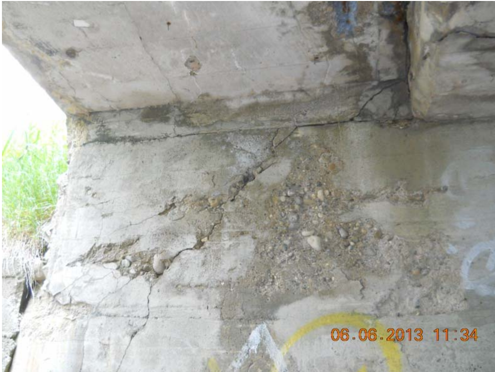
Delamination, spalling and scaling on abutment.
