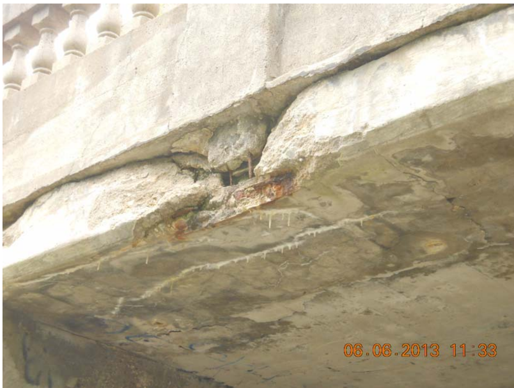
Spalls, exposed corroded rebar on fascia.
