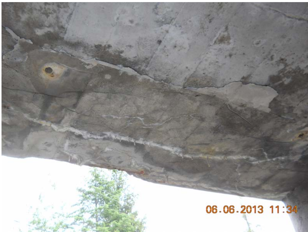
Delamination and efflorescence on soffit.
