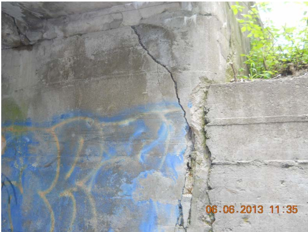
Wide crack on abutment.
