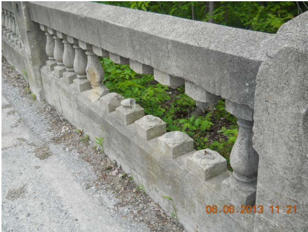
Missing spindles on barrier.
