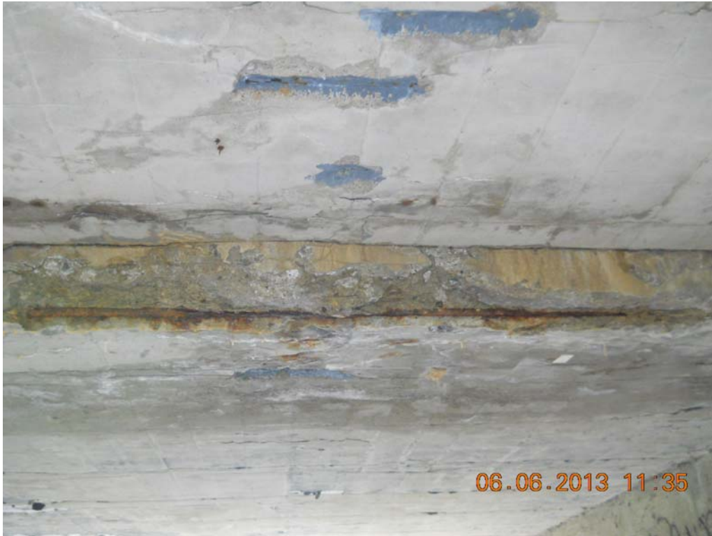
Delamination, spalling and exposed corroded rebar on soffit.
