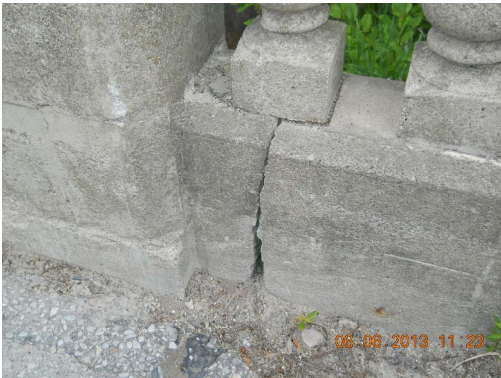
Wide crack on barrier.
